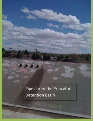
flowing directly into the valley area immediately to the west. Impounded water is collected at various locations and pumped into the NDC. Five pipes protruding from the south wall of the NDC mark the Princeton Detention Basin, maintained by the City, which is barely visible beyond the south wall. Water accumulating in the Basin is pumped into the NDC.
